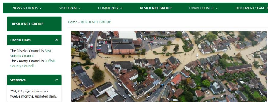
Framlingham Flood Resilience & Recovery
